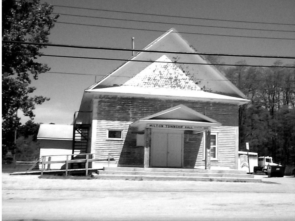
Old Milton Township Hall undergoing renovation, summer of 2003.
