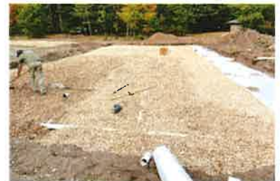
Barnes Park drain field replacement.
